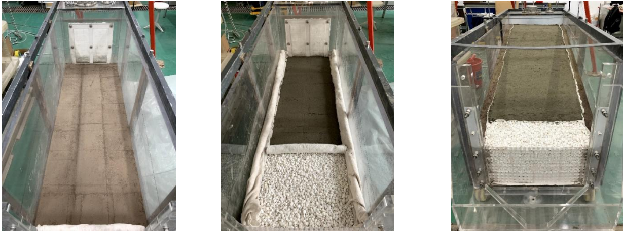
(a) Filling dam foundation (b) Filling tailings, initial dam, abutment (c) Dam slope ratio 1: 5
